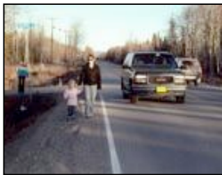
Plack Road in its current state
